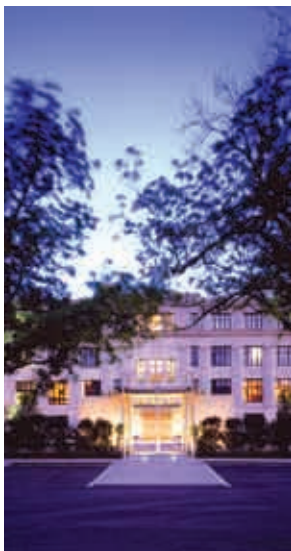
Photo Courtesy of Scott McDonald of Hedrich Blessing
