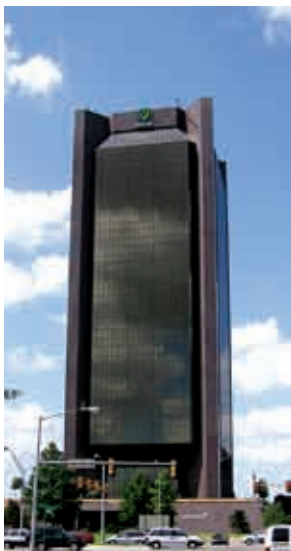
Photo Courtesy of Tom Gunning, AIA
