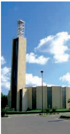
Photo Courtesy of Tom Gunning, AIA
