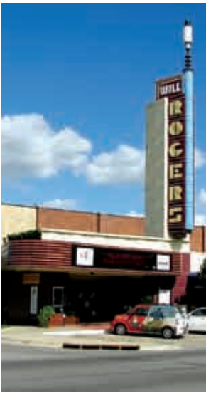
Photo Courtesy of Tom Gunning, AIA
