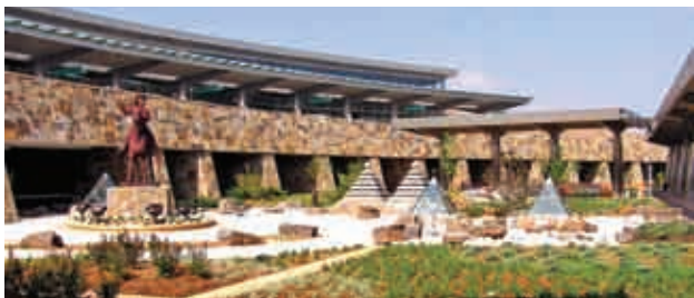
Photo Courtesy of The Benham Companies, LLC
